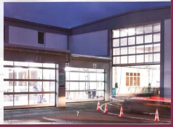
Sectional door SL in a car wash.
