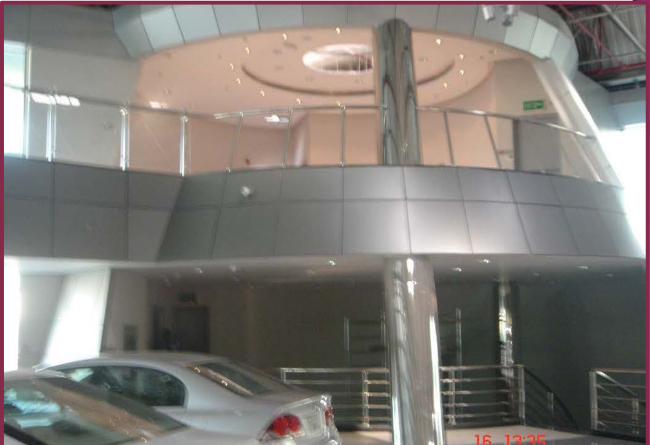
STAINLESS STEEL GLASS BALUSTRADE at KFH CARSHOWROOM - AL DHAJEED FARWANIYA Area
